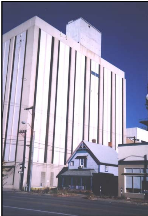
On Pikes Peak Avenue downtown, a home built in 1900 has as its neighbor a 1960s office building.
